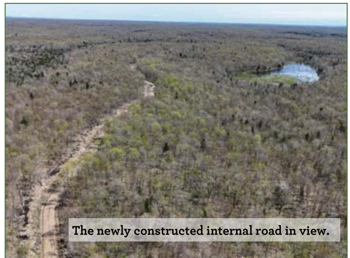
New internal access road through hardwood stand.
