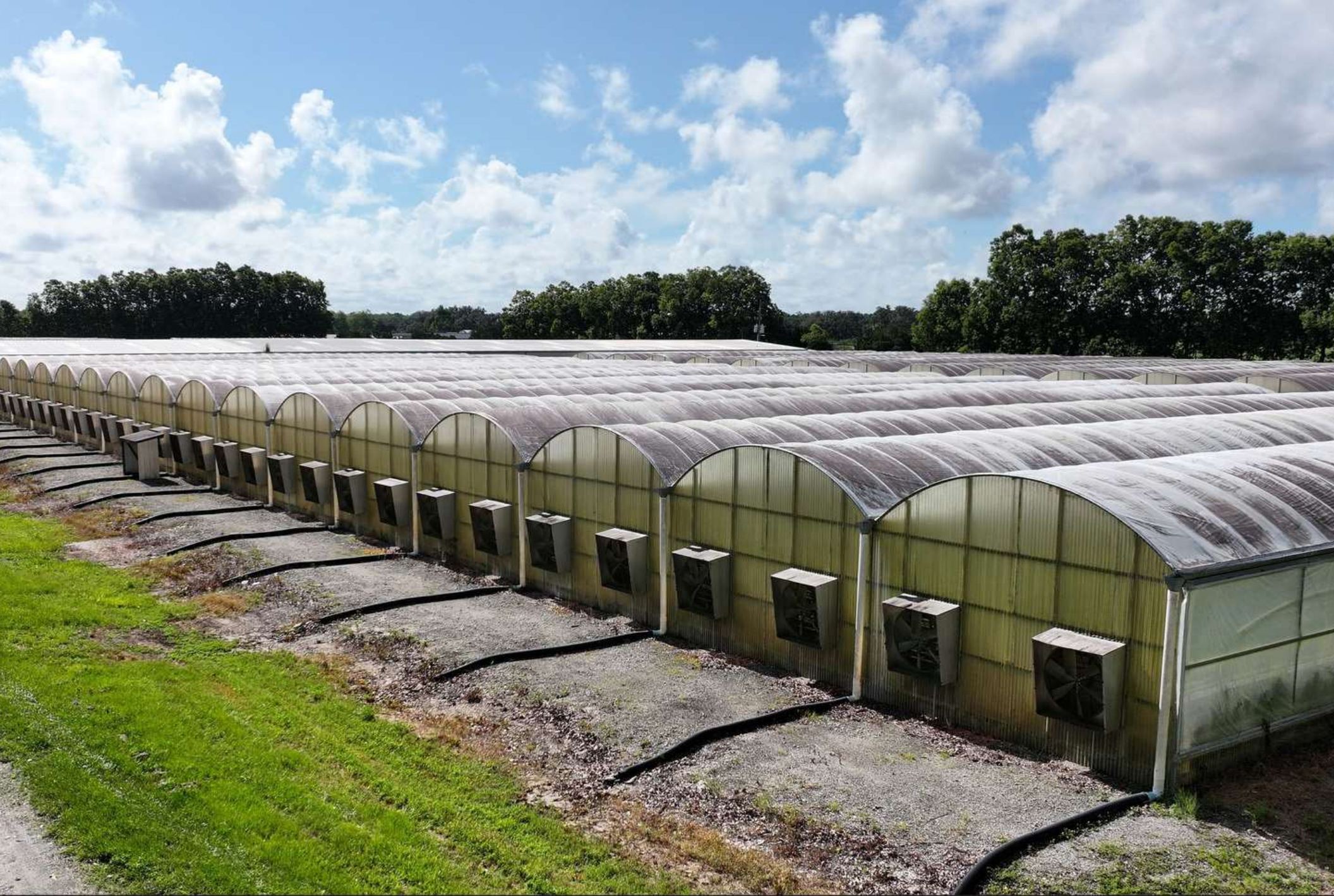
12 foot gutter height with 32 fans on each range of houses
