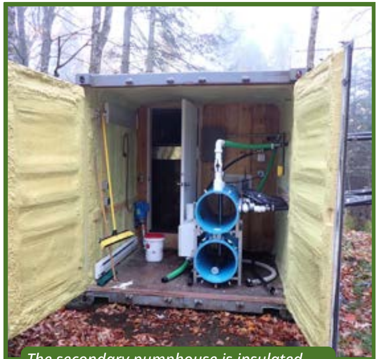
The secondary pumphouse is insulated and powered with electricity.
